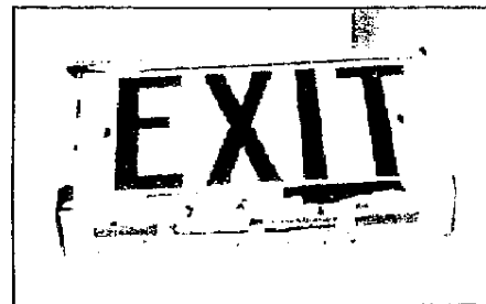
Exit light in a Vermont pool building rusted due to out-of-control humidity and a steel frame.
